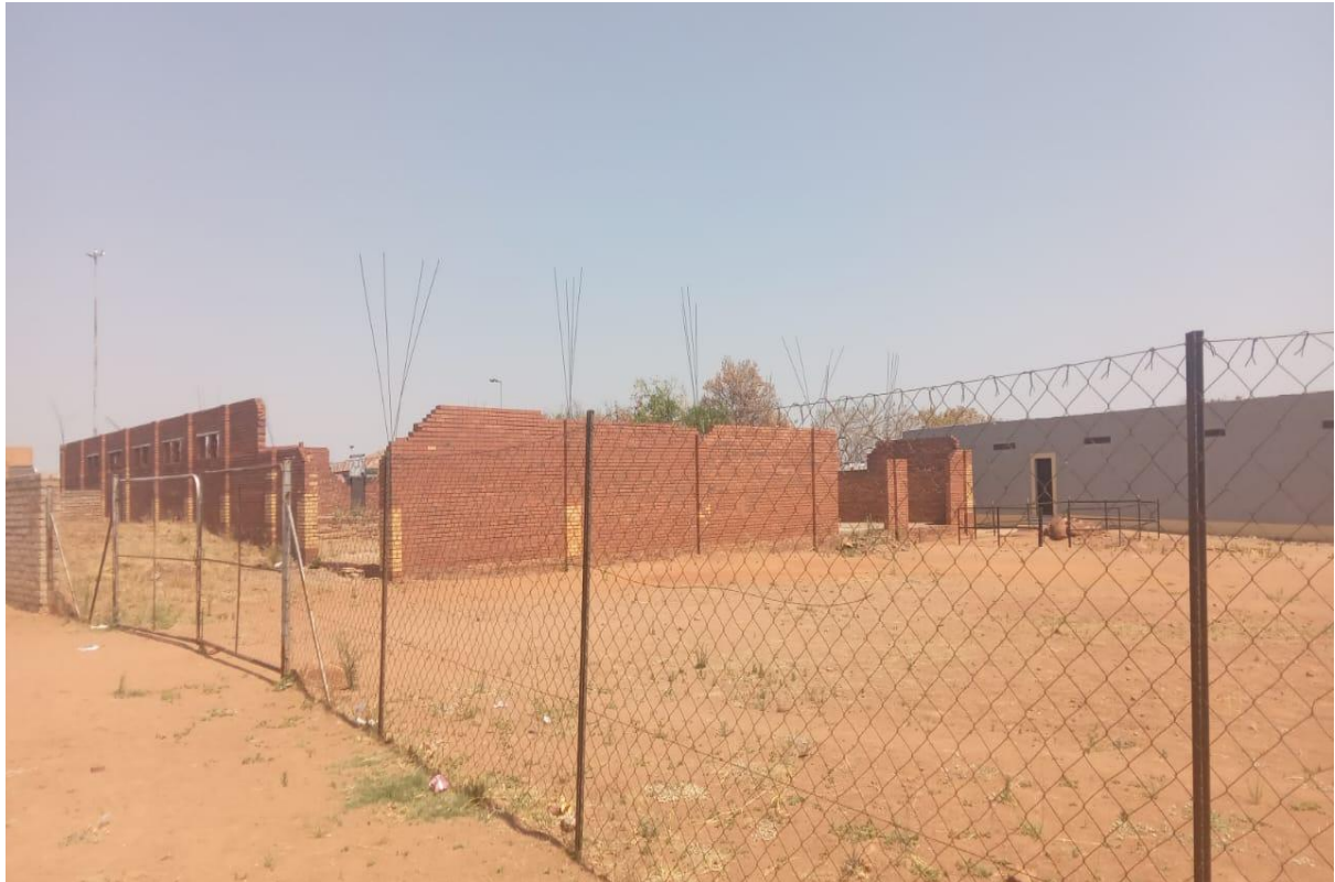
Figure 8: View of some of the structure noted on site.
